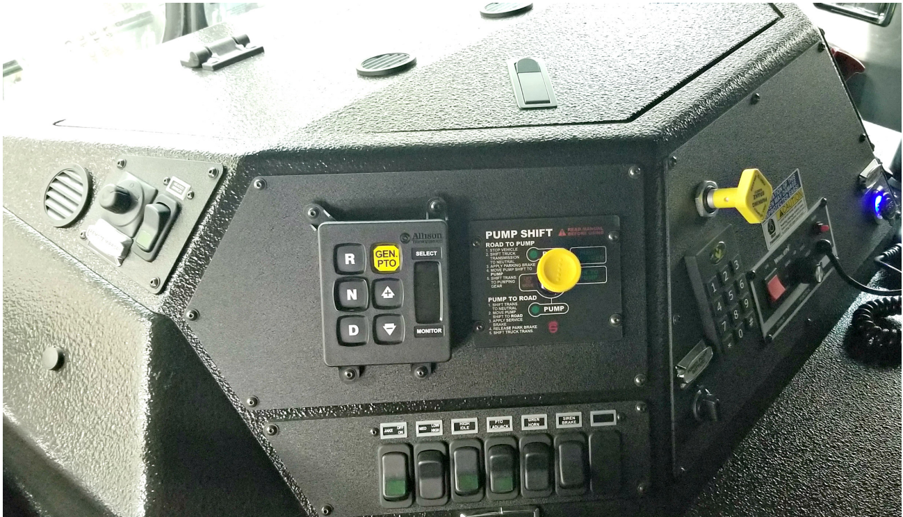
Mode Button (1) and Pilot Light (2) for Generator PTO
